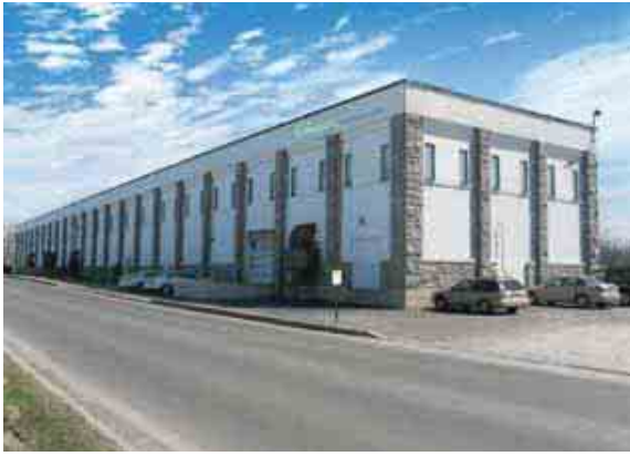
Drip Irrigation Systems : Jain Irrigation Inc., Watertown (USA)
