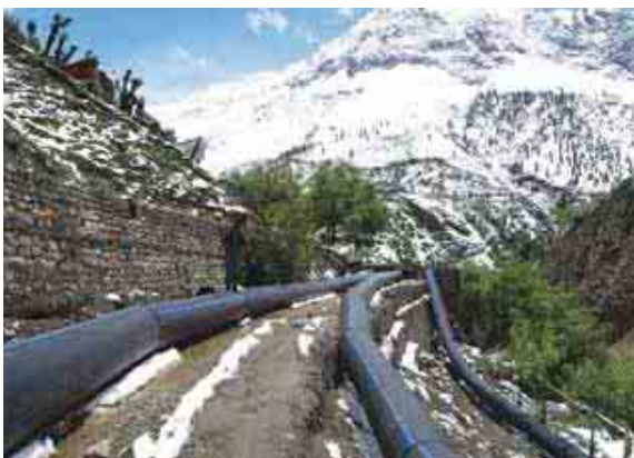
HDPE Pipe installed on the slopes of Himalayas
