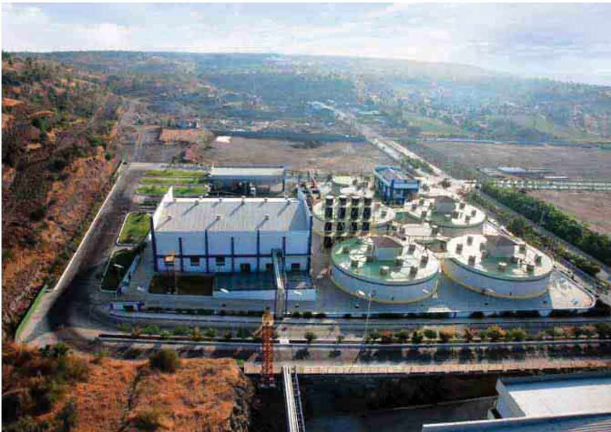
1.6 MW Bio-gas power plant
