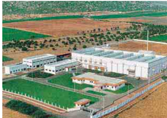
Drip and Sprinkler Irrigation Systems and Plastic Piping : Jain Agri Industrial Park, Udumalpet, Tamil Nadu, (India)
