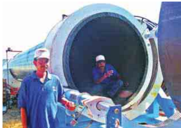
Installation of 1600 mm HDPE Pipe
