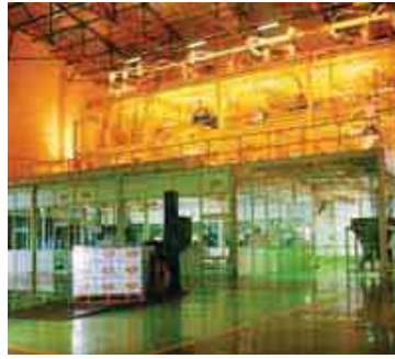
Onion dehydration facility
